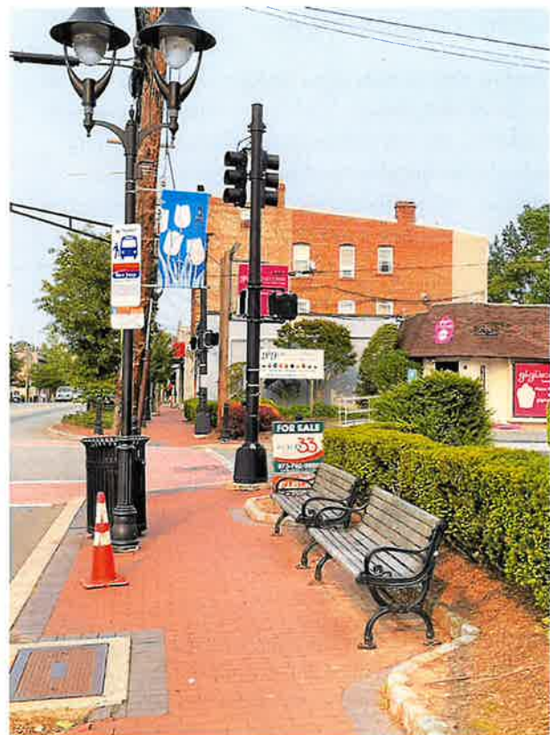
Existing Bus Stop along Springfield Avenue
