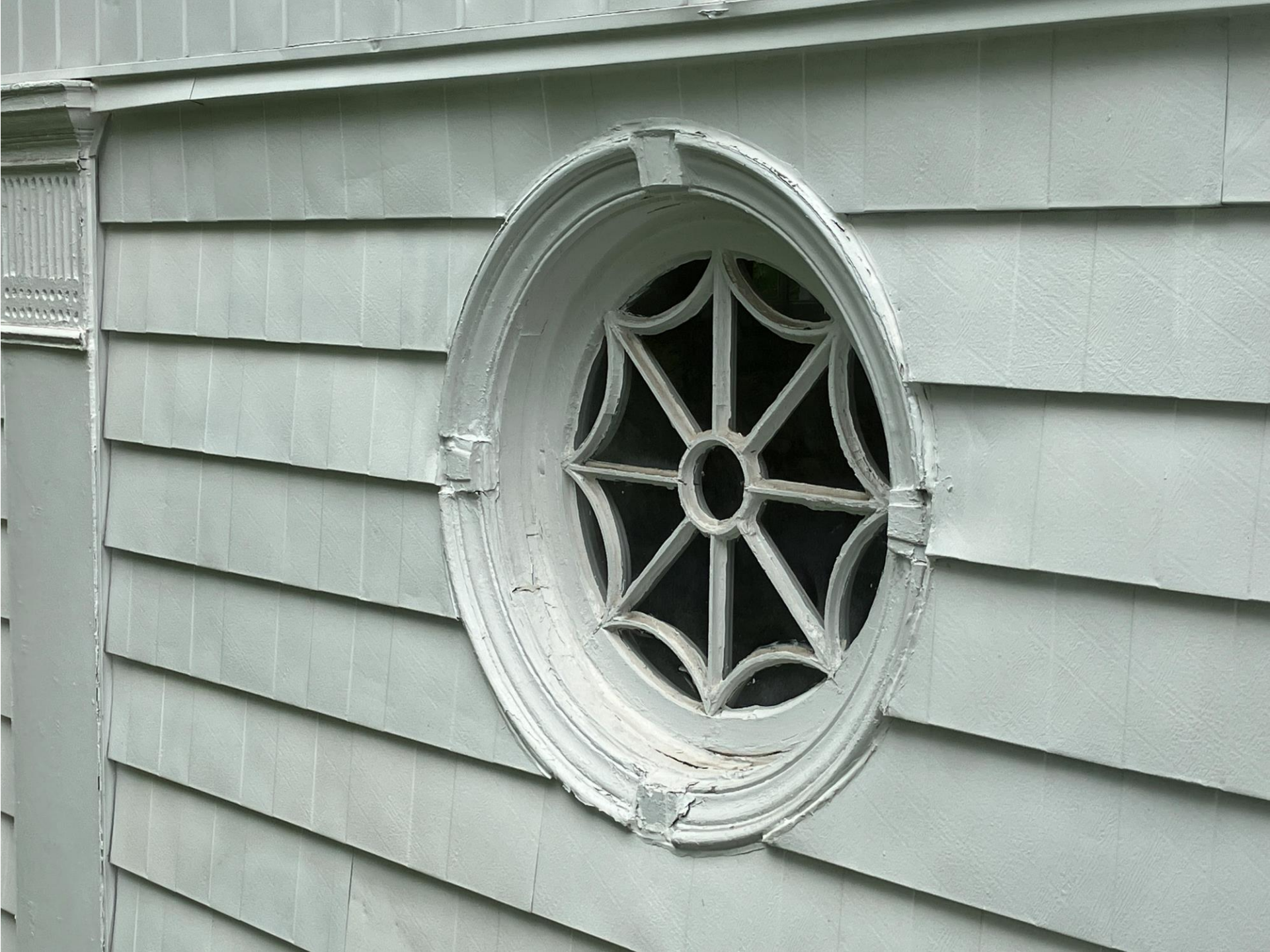
View of the rose window (W317); note the loss of definition in the detailing of the wood surround.
