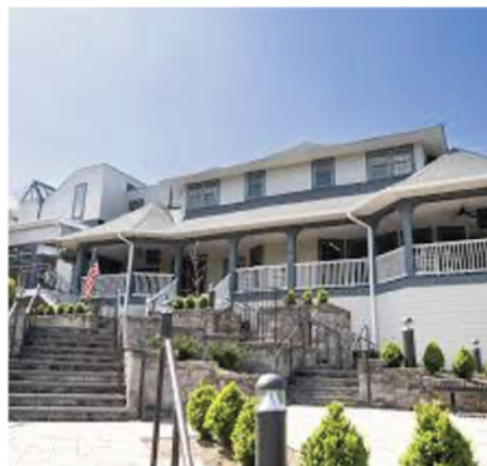
Image: Baird Community Center renovation and expansion
