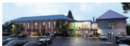
Library Building Connections Project featuring the renovated Connett building
